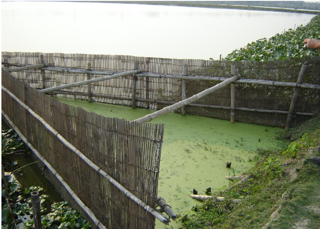
Picture 12. A bamboo screen filters solid waste from sewage before being brought into the fish farm
